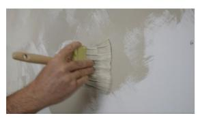
Apply 2 coats with a brush, mitten, glove or sponge with soft and rounded gestures or multidirectional patterns according to the desired effect, so that the paint load is not evenly distributed in order to the natural effect of the lime is enhanced and the water effect and shadows are accentuated.
